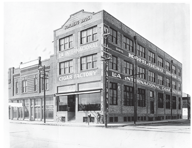
Kohlberg Bros. Cigar Factory is part of "People of the Crossing" documentary.
